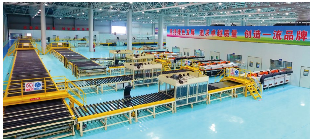
Triumph Science & Technology's New Energy Glass Production Base with One Kiln and Eight Lines
